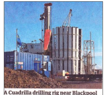
A Cuadrilla drilling rig near Blackpool
