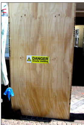
DANGER - unsafe building
