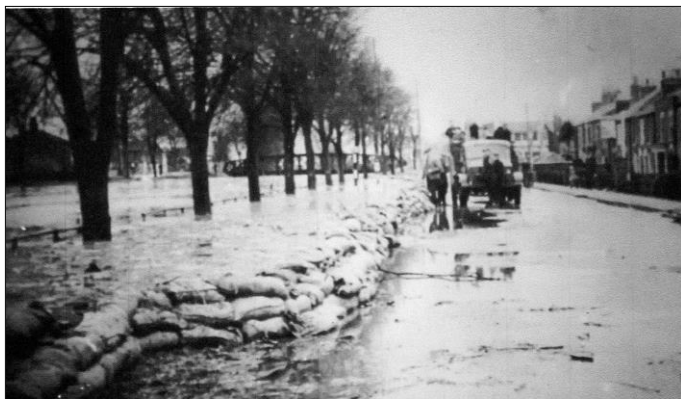
Flood water reaching the top of the sandbags in London Road
